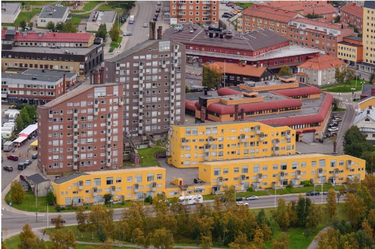
Figure 5.2: Kvarteret Ortdrivaren (aerial view).
