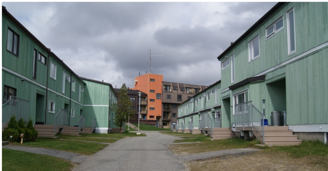
Figure 5.12: Above, wall South façade. Middle, wall North façade. Below, detached houses.
